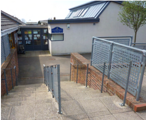
fig. View of Nursery Entrance.
